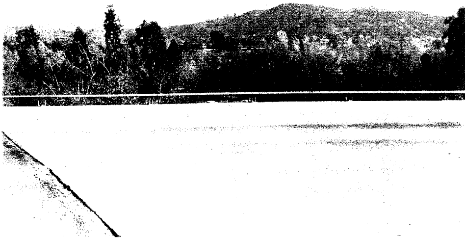
20. LOOKING UPSTREAM FROM CUYAMACA ST BRIDGE - CHANNEL TYPICAL SECTIONS 424 - 440 CHANNEL "N"= 0.05 - 0.075
