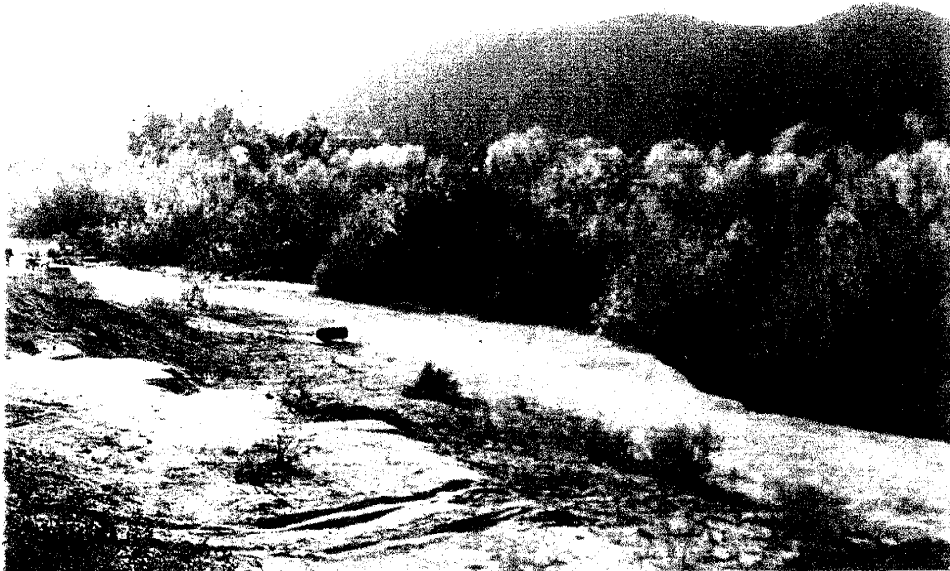
28. LOOKING DOWNSTREAM FROM RIVERFORD RD - LEFT OVERBANK TYPICAL SECTIONS 594 - 660 LEFT OVERBANK "N"= 0.75 CHANNEL "N"= 0.125 RIGHT OVERBANK "N"= 0.065
