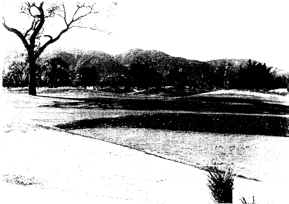
9. LOOKING DOWNSTREAM AT THE GOLFCOURSE - RIGHT OVERBANK TYPICAL SECTIONS 244 - 320 RIGHT OVERBANK "N"= 0.055
